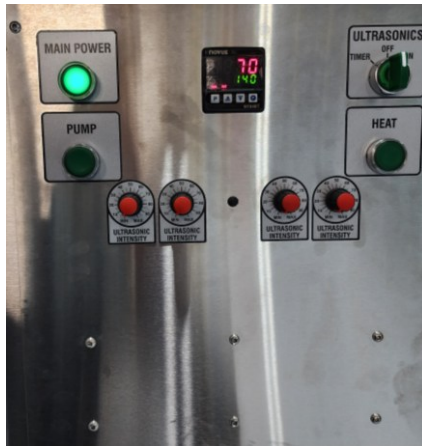
Figure 23 System Power On
