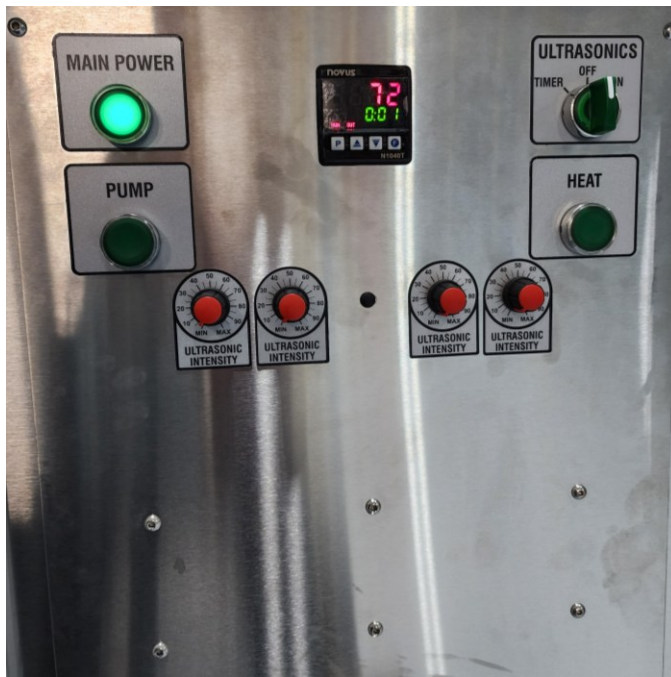
Figure 10 Generators Manual Control Off
