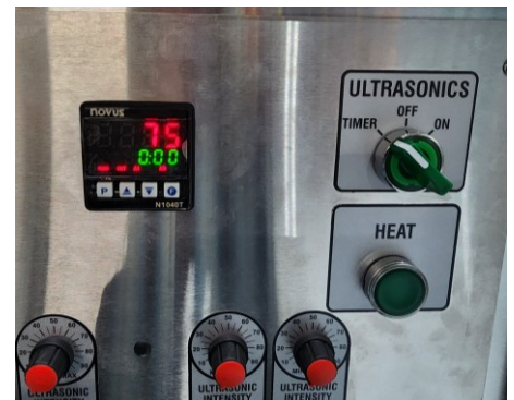
Figure 14 Generator Timer Cycle Done
