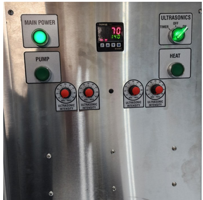
Figure 11 Generator Manual Control On
